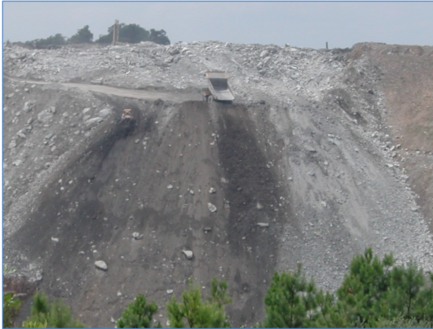
Figure 11. A valley fill in progress. (Photo courtesy of Vivian Stockman / www.ohvec.org )
